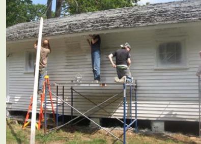
Movements Hall Repairs
